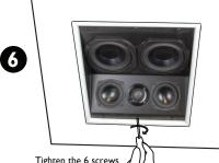
Tighten the 6 screws using a Philips screw driver so that the attached brackets securely clamp onto the ceiling/wall material (FXA550S shown).
